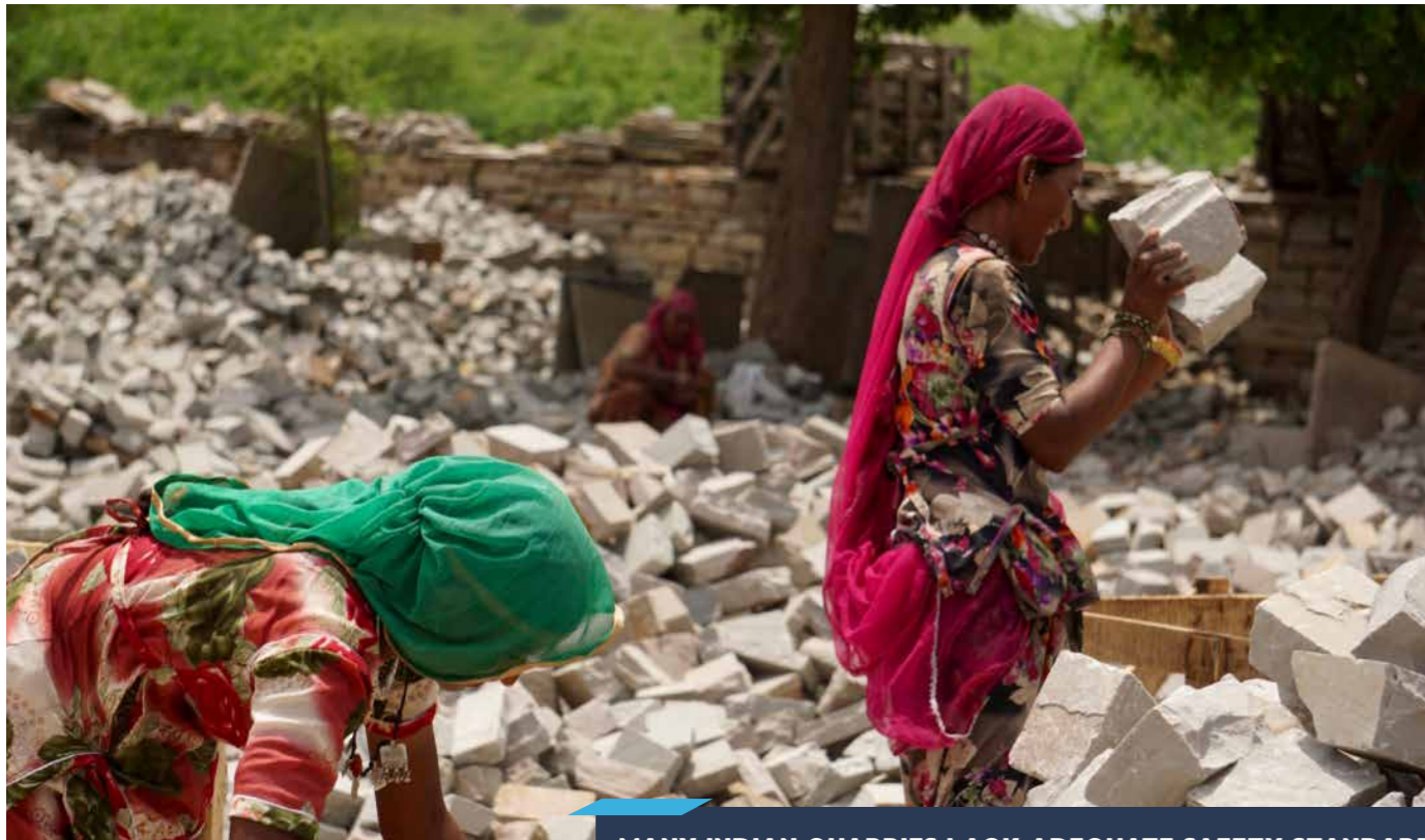
MANY INDIAN QUARRIES LACK ADEQUATE SAFETY STANDARDS.
